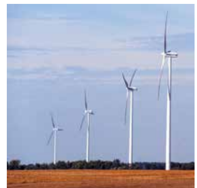
PSIcontrol ensures control of the energy generation.
