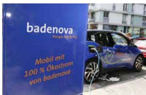
A smart charging station in the grid of bnNETZE.
