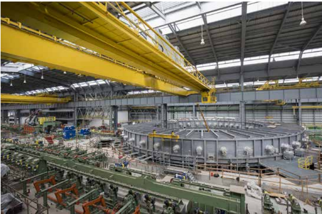
Construction of the rotary furnace in TenarisBayCity.
